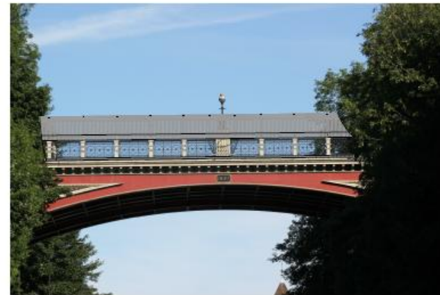
④ View From Road Below
